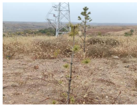
风机、箱变基础安装占地恢复植被
